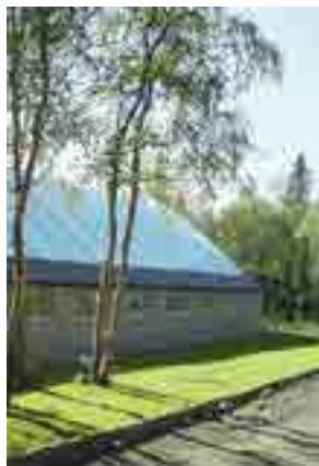
Greenhouse complex Photo by L.A. Ivanova
